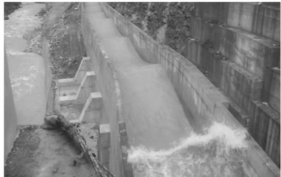
Figure 3. Water waves observed in the headrace channel of Nho Que 3 hydropower project ( $h = 9.0\text{m}$ ;  $b = 7.2\text{m}$ ), viewed from the intake
