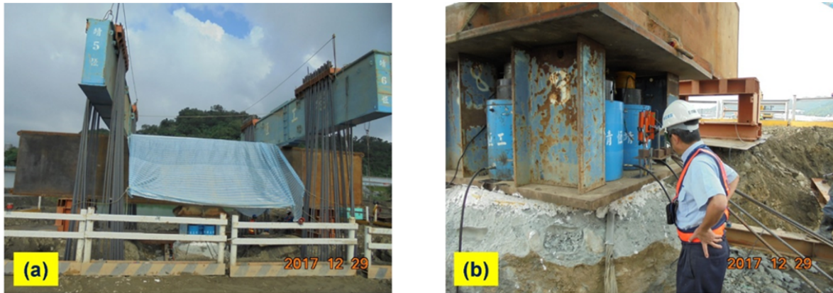
(a) Assembly of hydraulic loading system and reaction framework
