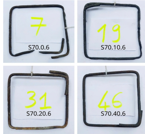
Figure 8. Surface of lateral reinforcing steel specimens after testing – Group 3 (6V)
