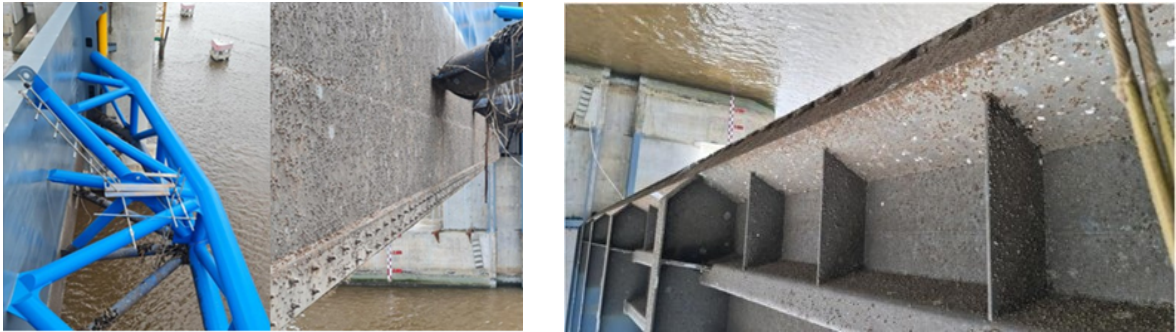
Figure 1. Biofouling on the sluice gates of the Cai Be project (two gates, 35 × 7.5 m)
