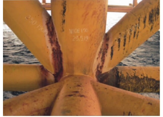
Figure 1. A corroded tubular joint on Jacket MSP 6 at the White Tiger field
