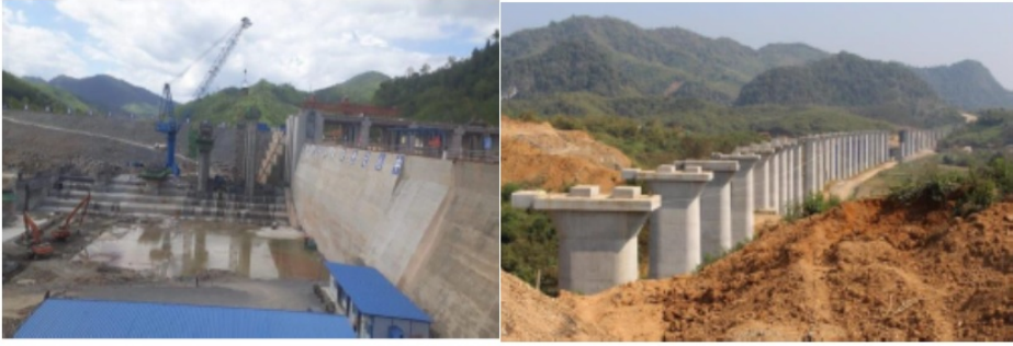
Figure 1. Application of fly ash concrete
