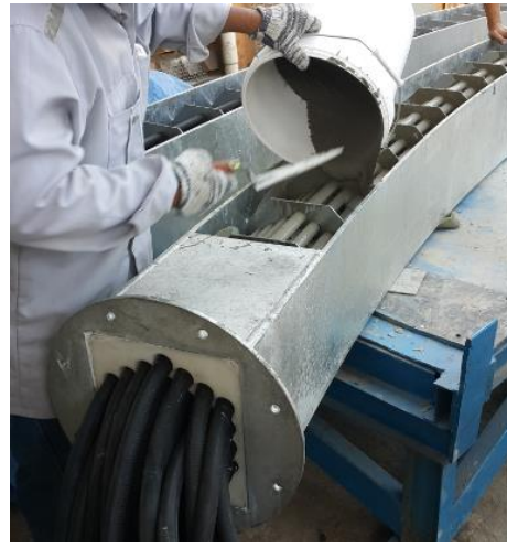
(b) HPFRC used for saddle anchor of extradosed bridge, Metro line 1, Ho Chi Minh city
