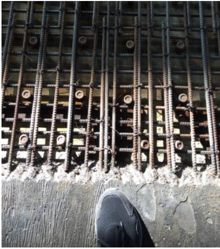
(a) HPFRC used for rehabilitating deck slab, Thang Long bridge, Hanoi
